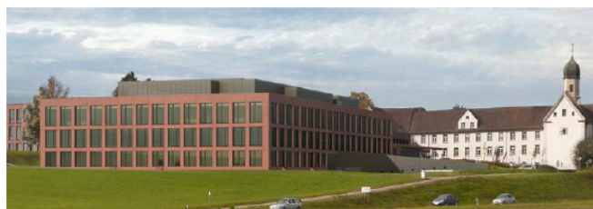
New »3i« building of the Münsterlingen cantonal hospital
